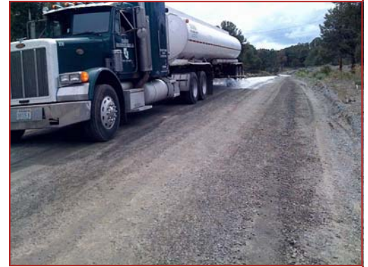
Application of Durablend Road Stabilization/Dust Suppressant Material
